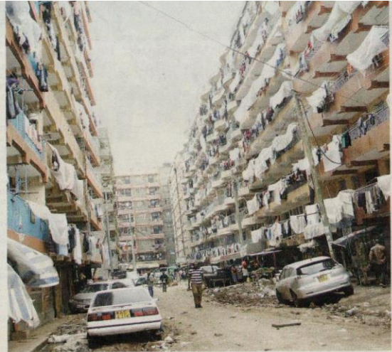
Some of the apartments in Pipeline estate. Most high-rise buildings have network problems. [File, Standard]
